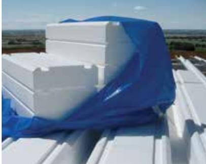
Fortruss is a forming system for insulated suspended concrete slabs. Light weight EPS deck panels are supported by metal clad truss forms that provide the formwork for suspended slabs. Applications include floors, decks and roof structures with clear spans of up to 40 feet. Pitched and sloped applications
