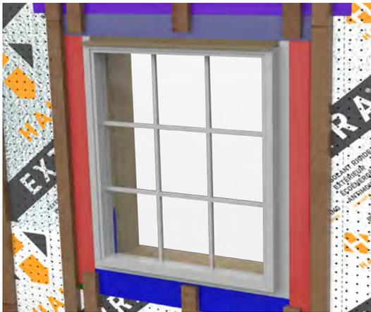
Step 8: Install trim boards and fasten to the furring strips or substrate.
